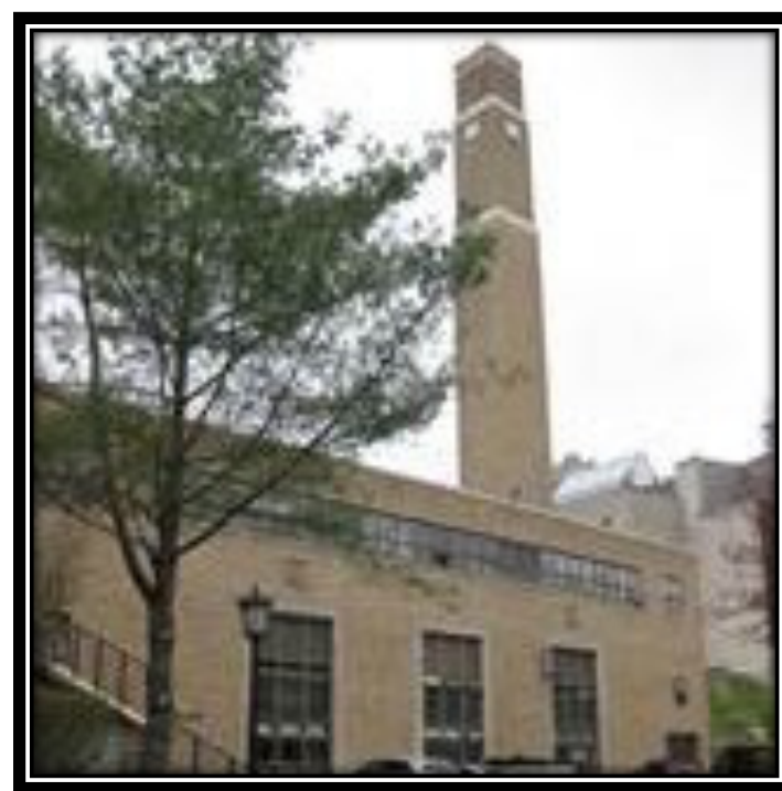
Figure 1: BC's Central Heating Plant powered by natural gas and oil (BC)
