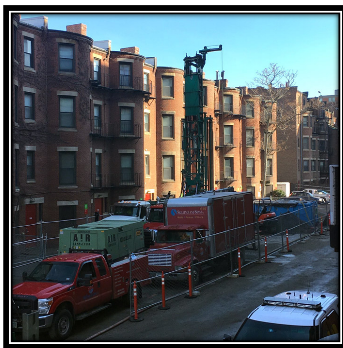
Figure 2: Drill rig at BU's new Data Sciences Center (BU)
