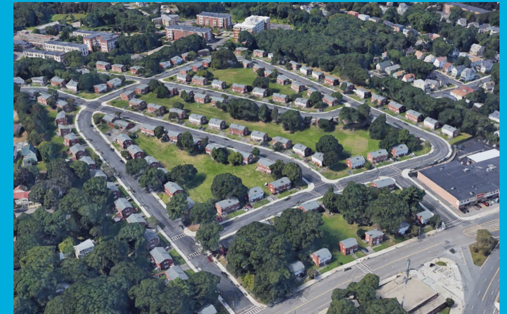
Gallivan Boulevard: An aerial view looking South towards Milton
